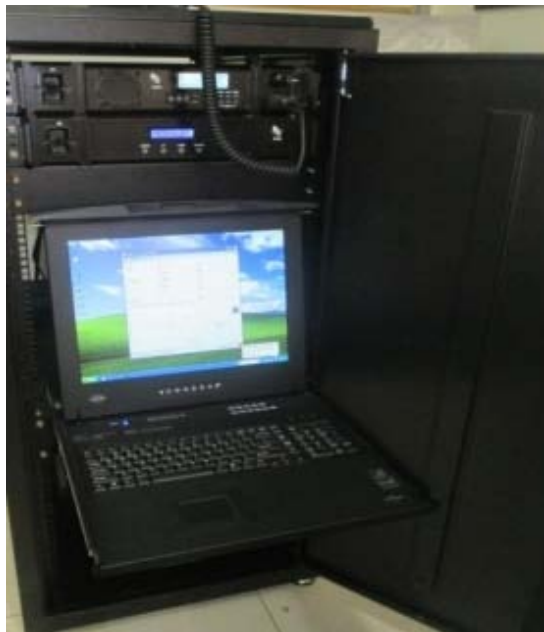
Gambar 5. Radio base station
